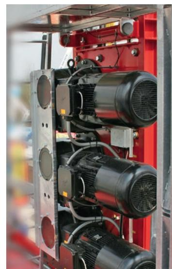
**Strong and safe.** – Electronically controlled geared motors gently move loads of several tons.
