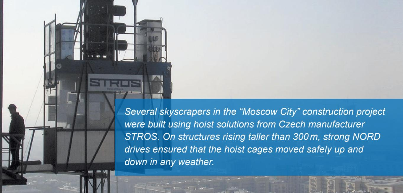
Several skyscrapers in the “Moscow City” construction project were built using hoist solutions from Czech manufacturer STROS. On structures rising taller than 300 m, strong NORD drives ensured that the hoist cages moved safely up and down in any weather.
