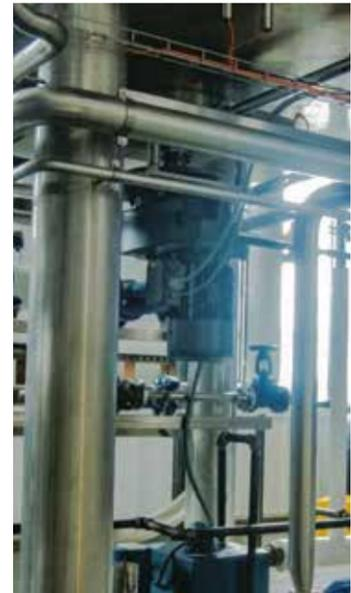
A 5 hp Parallel shaft gear unit powers the rake in the Mash Tun.
