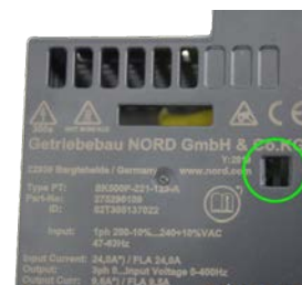
Frequency inverter without STO contact jumper
