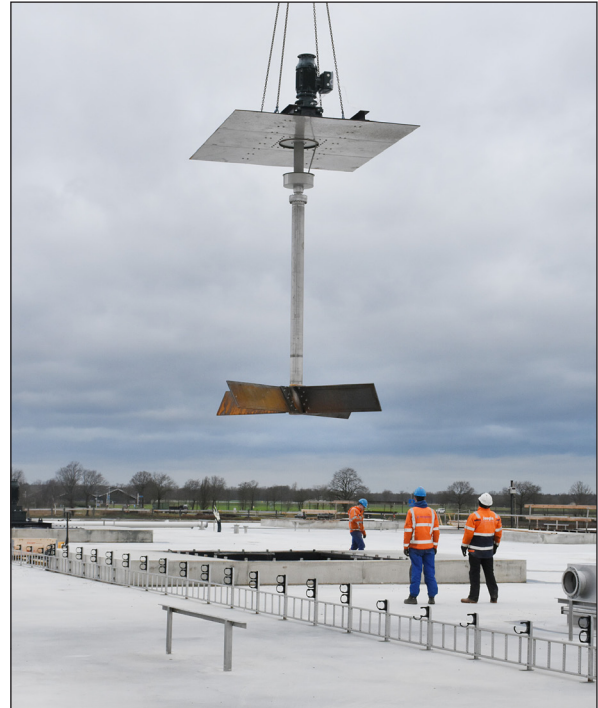
Right: The agitators are lifted to the roof of the fermentation plant by a crane.
