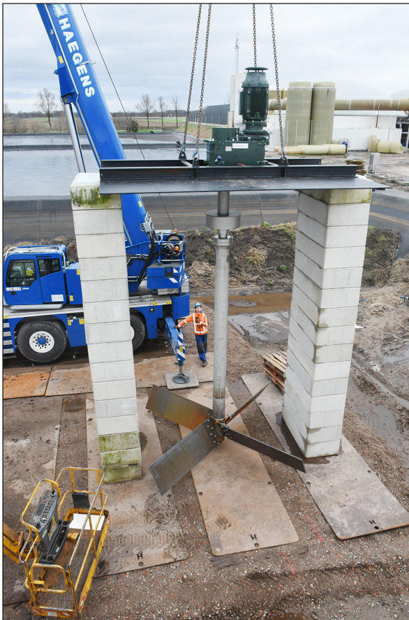
The agitators were assembled on site...
