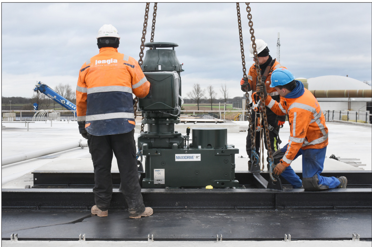
Below: Technicians ensure that the agitators end up in exactly the right place.
