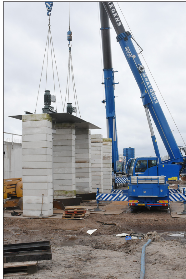
...and lifted into place with a crane.
