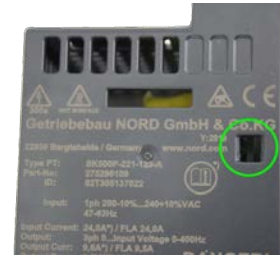
Frequency inverter without STO contact jumper
